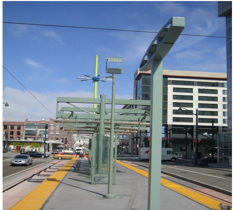
Existing Fourth & King Station (Typical)
